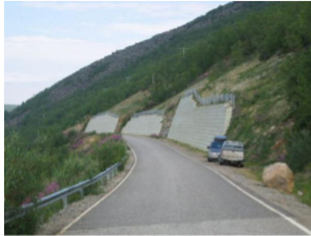
A rock wall stabilizes a slope that has been cut away to make a road. Retaining walls in Finland Utsjoki by Timo Saarenketo, https://lic.kr/p/edQe41 , CC-BY
